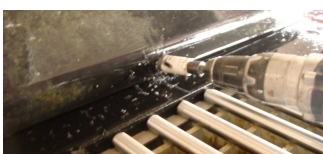
37 mm hole for injector hose
